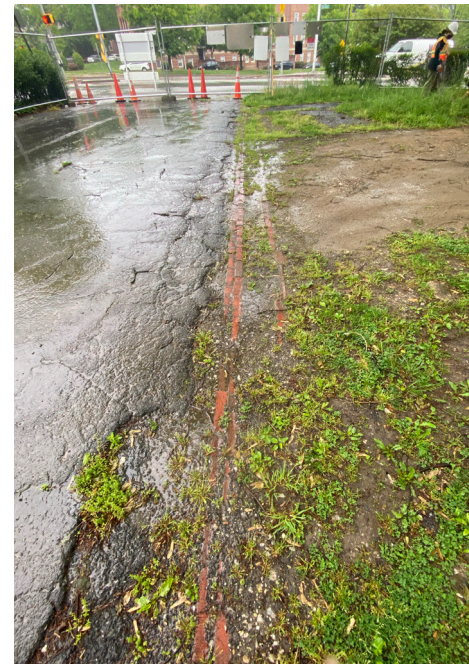
Roadway Condition Details - Concrete Curb at inner edge; Brick & Concrete Runnel at outer edge
